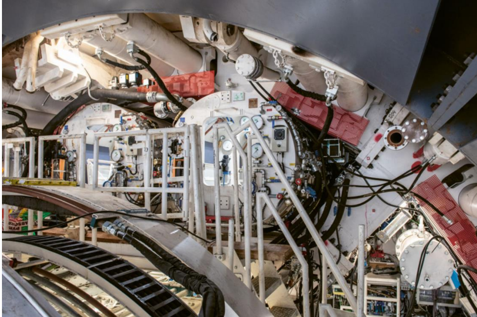
Photo credits Implenia - Tunnel boring machine Metro Line B - Lyon
